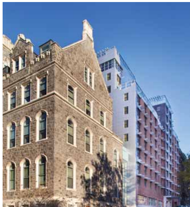
Fortune Society's Castle Gardens in West Harlem: 113 apartments for a mix of formerly homeless and low-income families and singles.
