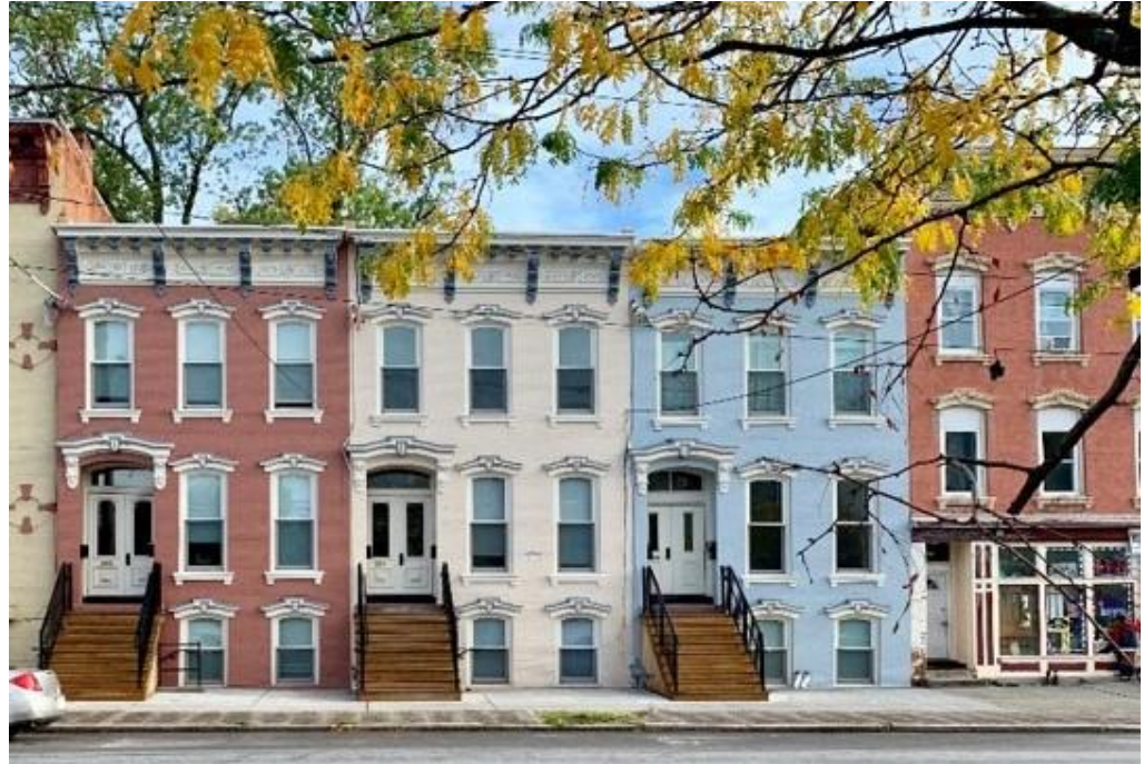
Clinton Avenue, Albany
